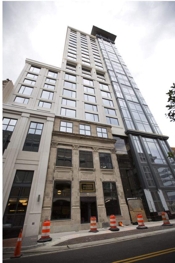
L. Todd Spencer | The Virginian-Pilot Photos of the historic Decker facade, restored at The Main Hotel and Conference Center downtown Norfolk, Jan. 29, 2017.
